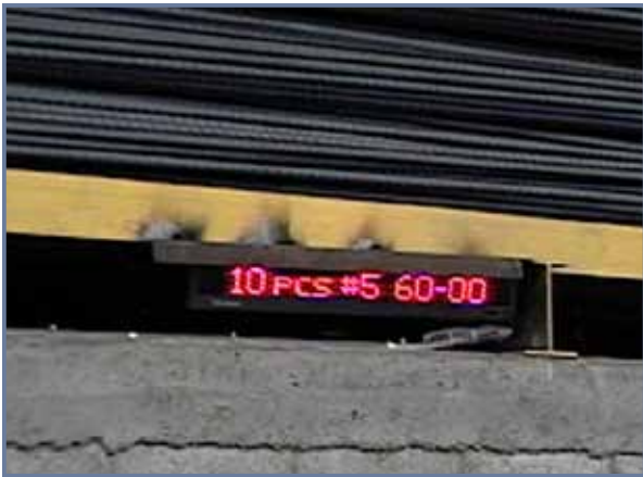
aSa's console does more than control the shearline. It provides a thorough production plan for the entire shop crew. For example, a message board connected to the console tells the shake-out person what stock is required next.
